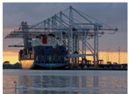
Ship to shore cranes.
