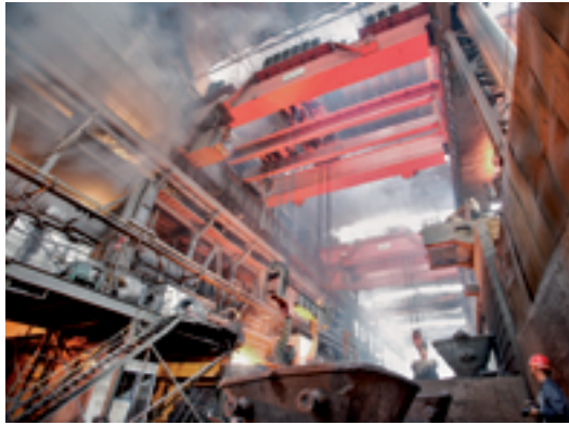
Travelling crane in steel plant.
